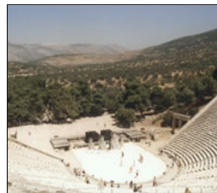
Modern actors can be heard clearly 60 metres away on a windless day.
